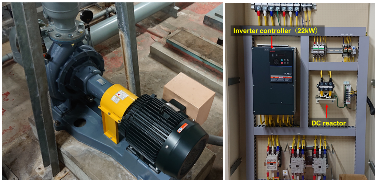
Fig.1. (left) newly installed pump, (right) inverter circuit
